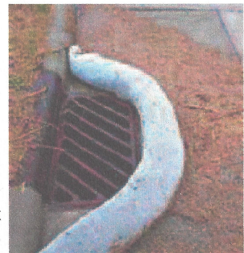
A compost filter sock protecting a storm drain.
